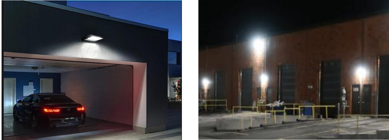
Fig. 32.04.07-B: Wall pack lighting with cut-off (left) and without (right)
